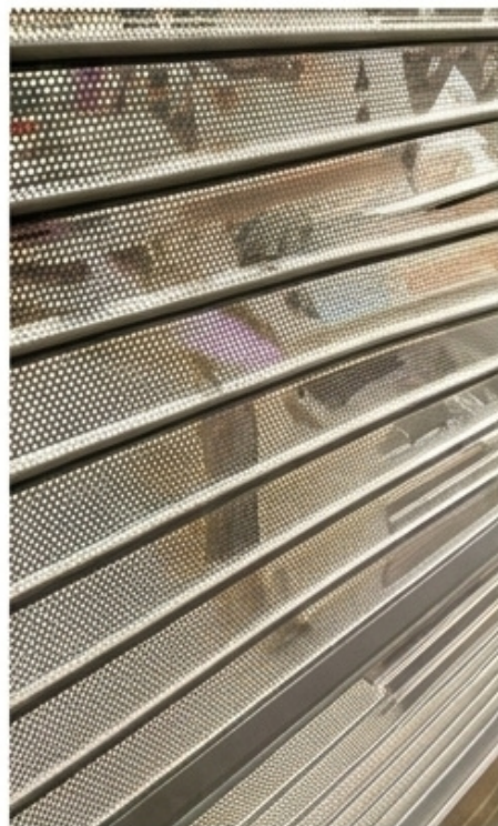
Detail of 40% Perforation (3mm Dia)
